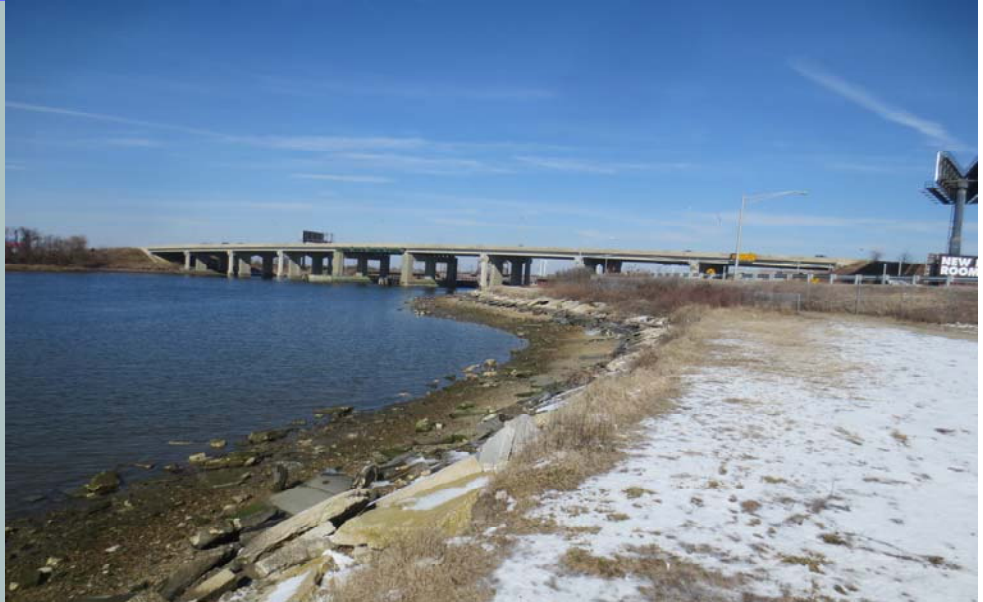
The area near sunset avenue in Atlantic City is protected by a low poorly constructed rubble revetment that is easily overtopped by storm surge during flood events
