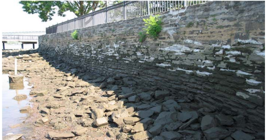
View of seawall with recent local repairs
